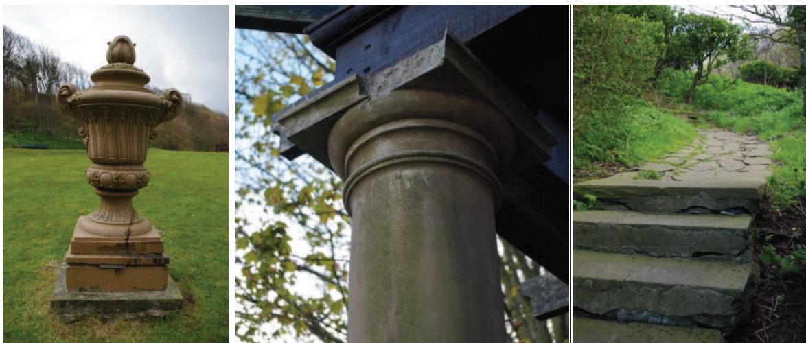
Plate 54. Fractured ceramic urns, spalling concrete structures and decaying steps of stone and concrete present substantial conservation requirements.
