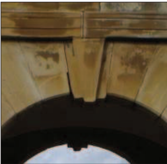
Plate 60. Several stone structures while in reasonable condition require scheme of repointing and minor repair to forestall more major decay.
