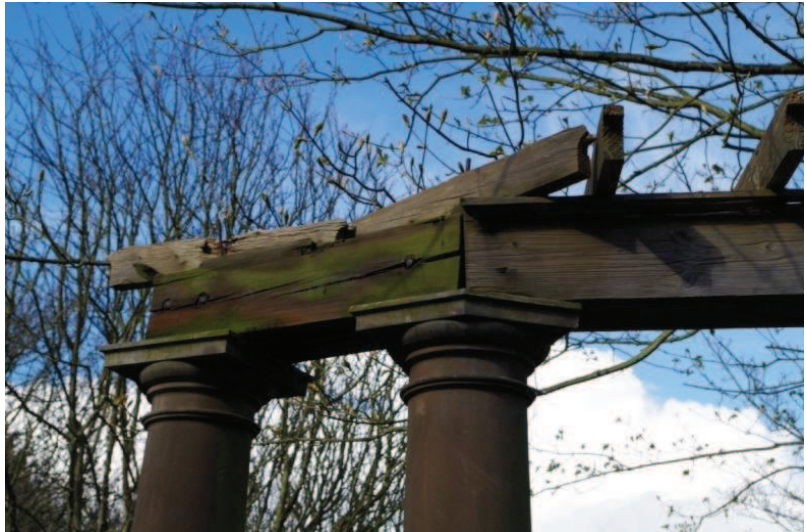
Plate 55. Many of the wooden shelters/arbours, some of 19 th century date have been restored in the last 20 years. Despite maintenance the harsh marine environment means timber continues to decay and needs further attention seen in rotting bases (above left), damaged and decaying pergolas (above right), distinctive ceramic tile shingled roofs (below left) and internal tiled floors (bottom right)
