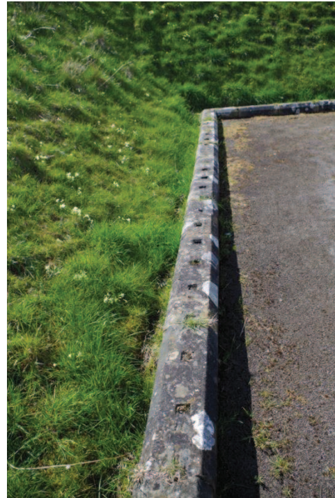
Plate 58. Damage to the Italian Steps, missing features, spalling stonework and subsidence with no formal planting
