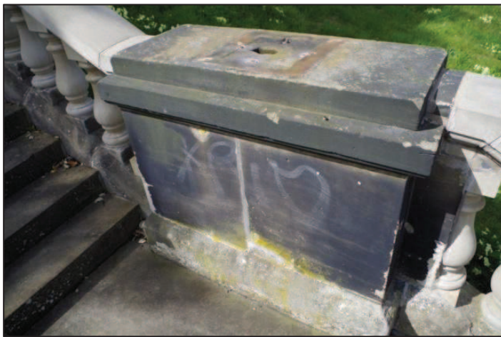
Plate 58. Damage to the Italian Steps, missing features, spalling stonework and subsidence with no formal planting
