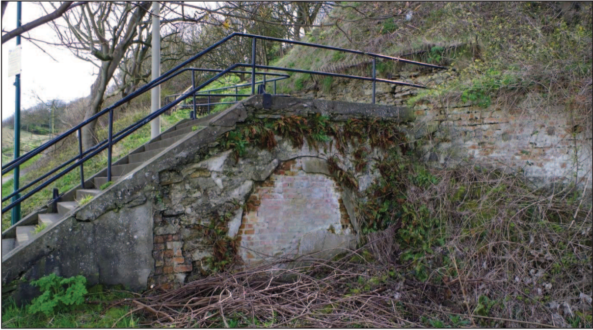
Plate 18. The pedestrian tunnel beneath the Cliff Railway of 1875. (Above) looking south as it goes beneath the steps parallel to the railway; (below) the finer quality stonework as the tunnel goes under the railway itself showing a slipped voussoir, single skin brick blocking and negative modern features of chain link fencing, metal steps and lighting. The area between the two tunnels was at one point covered by a small building (see plate 17).
