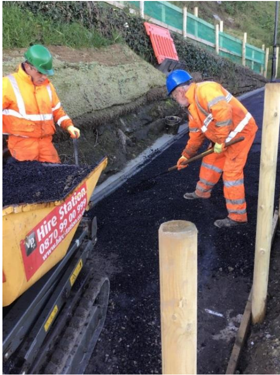
Footpath surfacing works.
