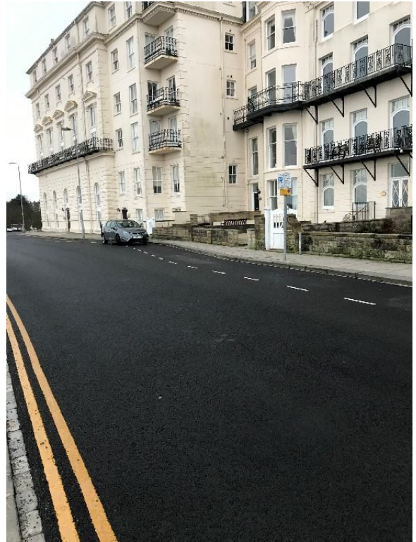
Newly laid tarmac on The Esplanade.
